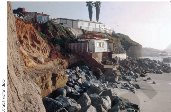
► FIGURE 13-50. Collapsing sea cliffs at Ocean Beach near San Diego destroyed some homes and severely threatened those remaining in March 1998. Huge boulders were placed at the base in an attempt to arrest the erosion.
