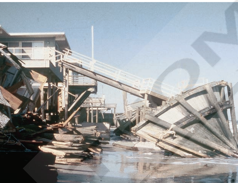
► FIGURE 13-16. The Nor'easter of December 29, 1994, undermined this vertical steel wall at Sandbridge Beach, City of Virginia Beach, Virginia, and toppled into the surf.
