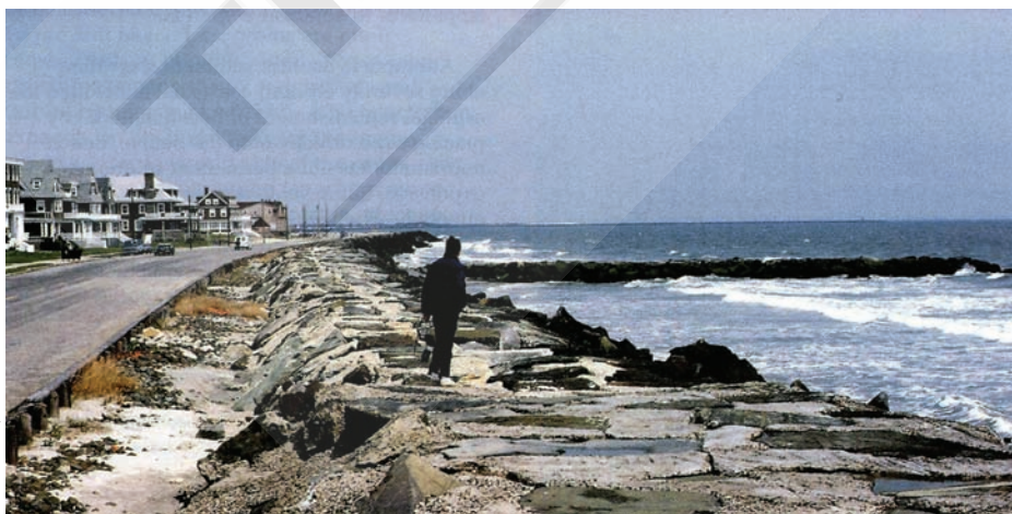
► FIGURE 13-27. This is the sad ending for a mishandled beach at Cape May, New Jersey. The building of jetties at Cape May Inlet just up the coast trapped the sand that previously replenished the beach. A concrete and rock seawall now lines the “beach.”
