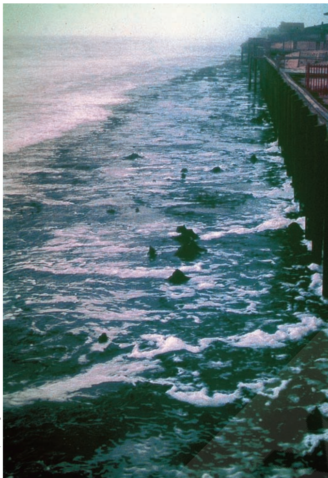
► FIGURE 13-43. Peat blocks and stumps in the surf at Sandbridge Beach, City of Virginia Beach, originally formed in the lagoon behind the barrier island decades ago. The island has since migrated landward over the lagoon. Note the imposing wall supposedly protecting buildings from the waves.
