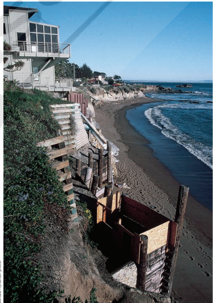
► FIGURE 13-52. Timbers were installed in an attempt to protect an eroding beach cliff below houses in Pismo Beach, California.
