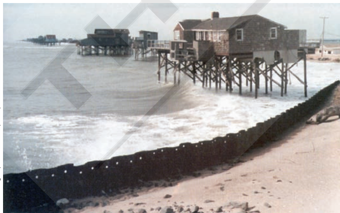
► FIGURE 13-41. Storm waves reduced the level of sand by almost 4 meters during one storm at Westhampton, New York. The barrier island migrated landward, leaving these houses stranded offshore.
