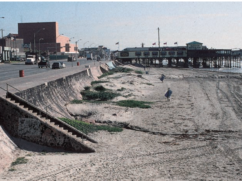
► FIGURE 13-15. The massive seawall at Galveston, Texas, was built after the catastrophic hurricane of 1900. Beach sand eroded by waves at the base of the seawall is continually replaced by truckloads of sand brought in from coastal dunes.
