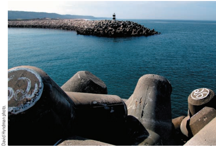
► FIGURE 13-14. These huge interlocking concrete pieces are designed to reduce wave energy and protect the harbor at Nazare, Portugal.
