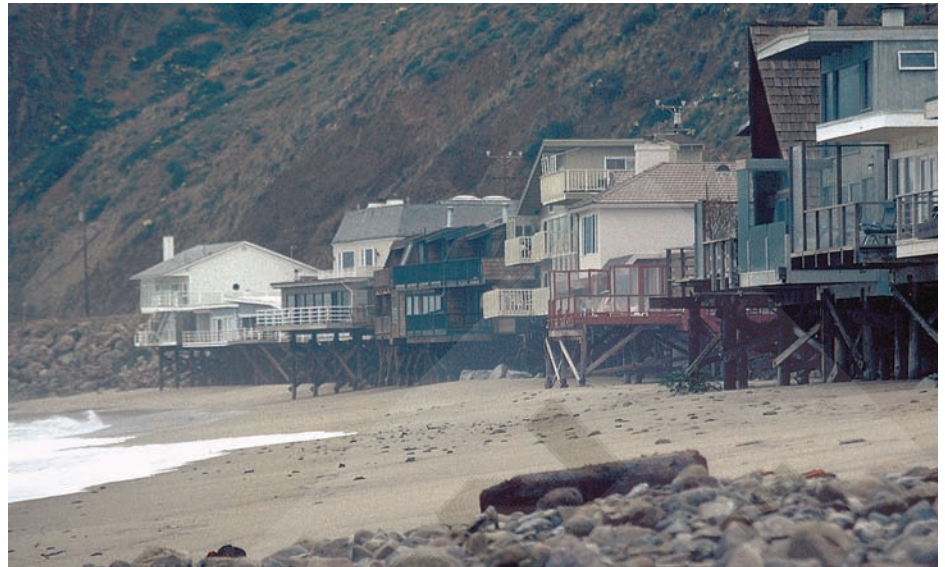
► FIGURE 13-53. These homes were built on pilings on the beach west of Malibu, California.
