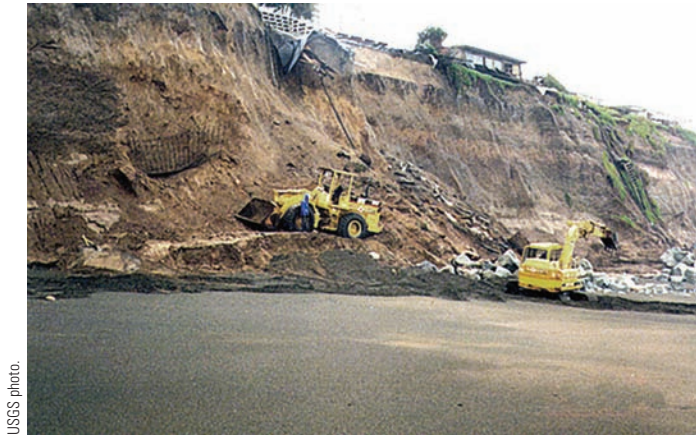
► FIGURE 13-49. Heavy equipment tried desperately to pile heavy riprap boulders at the base of the same rapidly eroding cliff shown in Figure 13-48 before the next high tide in January 1998. Note the house debris at the base of the cliff.
