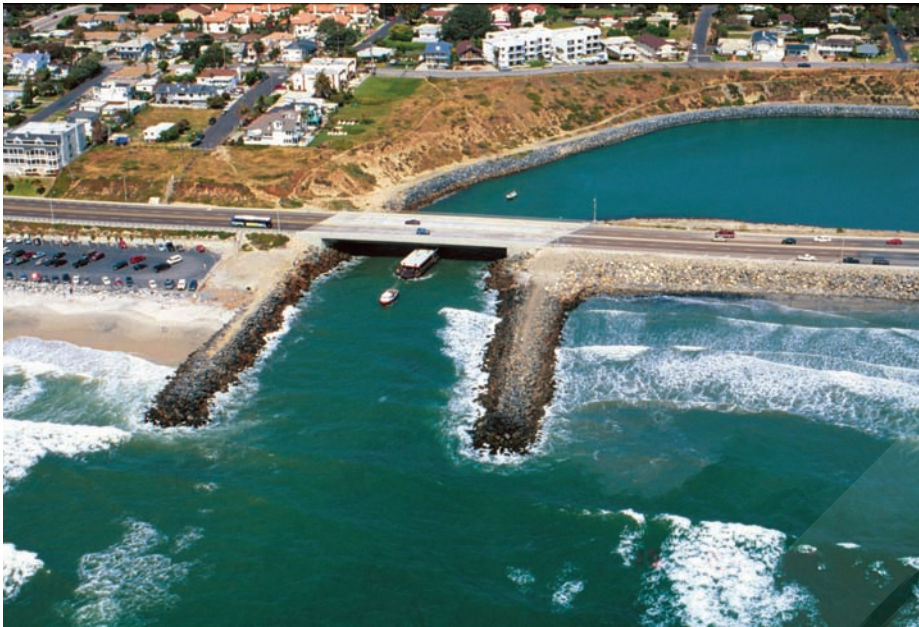
► FIGURE 13-21. Longshore drift is interrupted at jetties just as it is at groins. The beach on the right side of this jetty north of San Diego has been completely eroded by longshore drift of sand from left to right.
