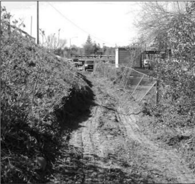
Figure 1. A newly bulldozed construction site provides a transient opportunity.
